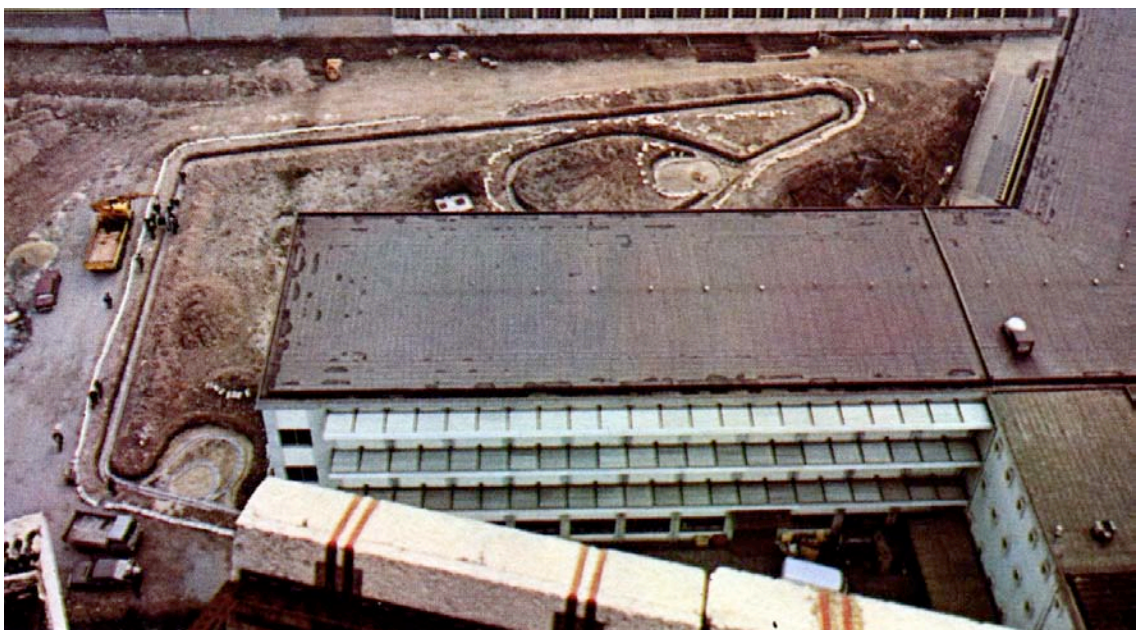
Fig. 3 – Cable trench during laying 1
